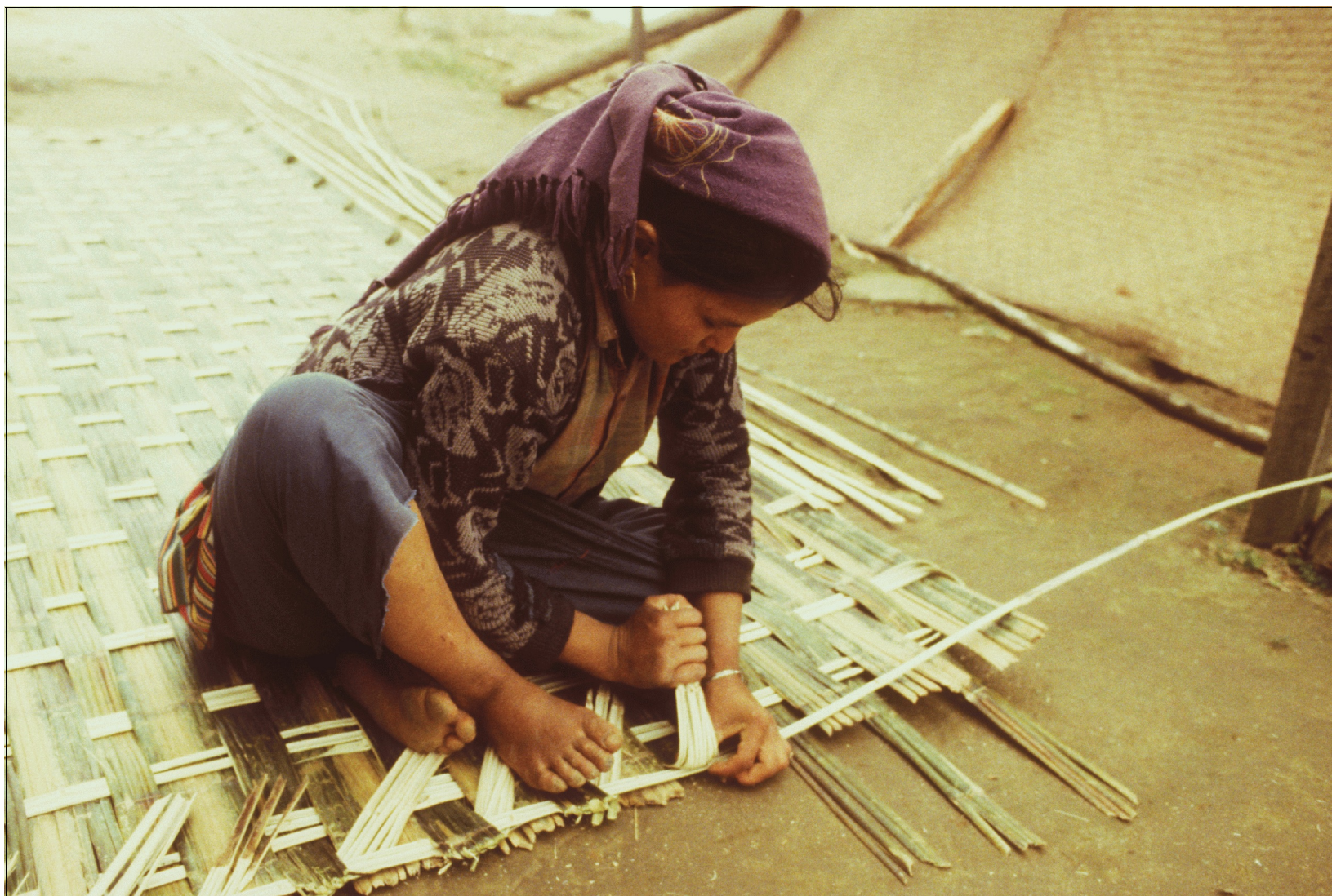
FIGURE 2.21. Woman weaving a chitra panel from split malingo bamboo, which will be used to construct or repair the wall or roof of a traditional home or livestock shed.
